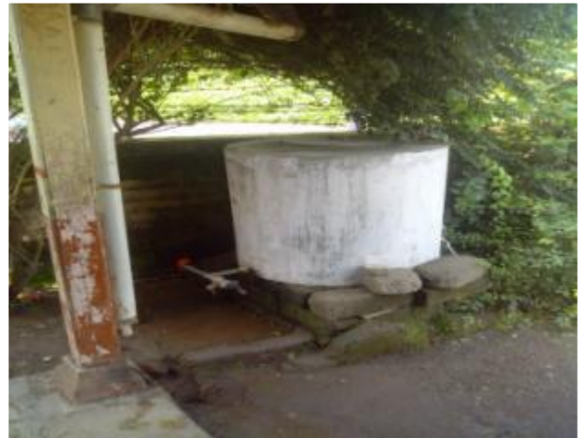
Water tank at Rethvaniya PS
