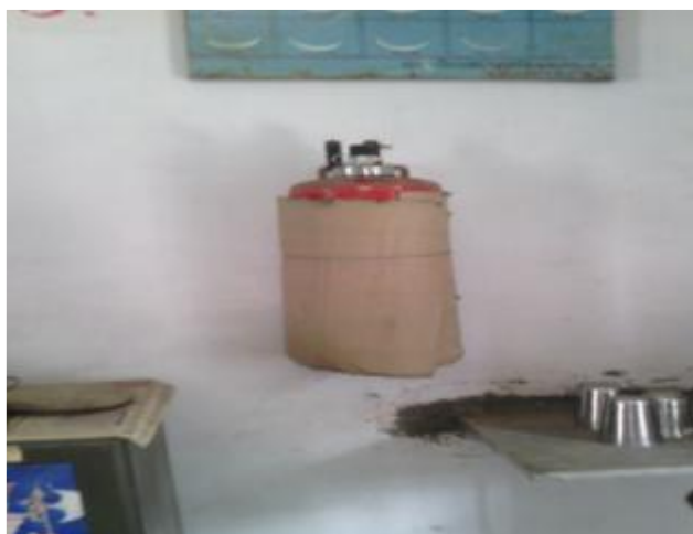
Fire extinguishers placed in kitchen at Vir Mangal Pande PS
