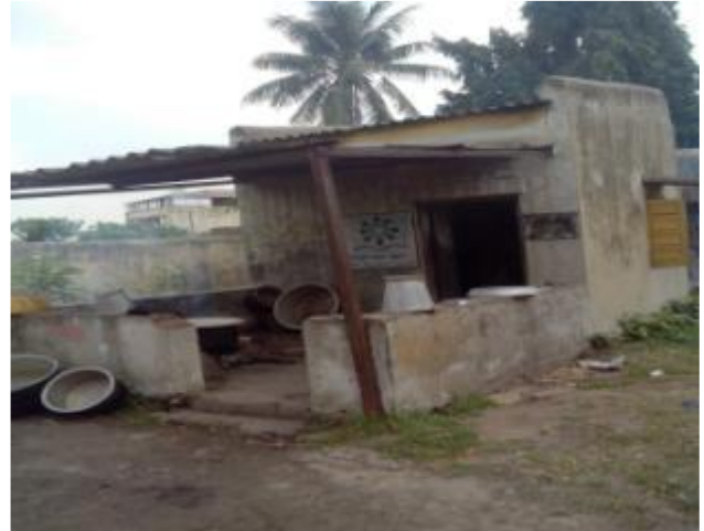
Old kitchen shed found at Kanav PS
